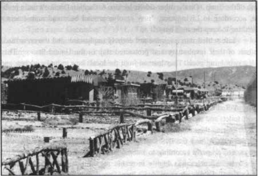
Cottages constructed by German internees at Fort Stanton (Courtesy of Werner Prager, Jr., and the Lincoln County Heritage Trust)
