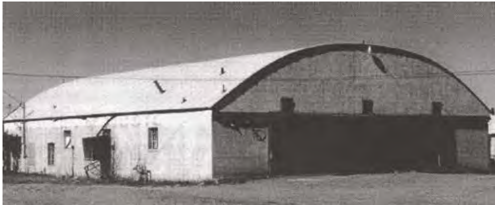
New Mexico College of Agriculture and Mechanic Arts, Hangar
