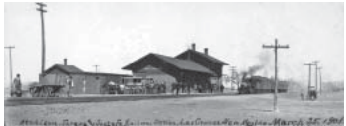
Atchison, Topeka and Santa Fe Railway Station, Las Cruces, NM
