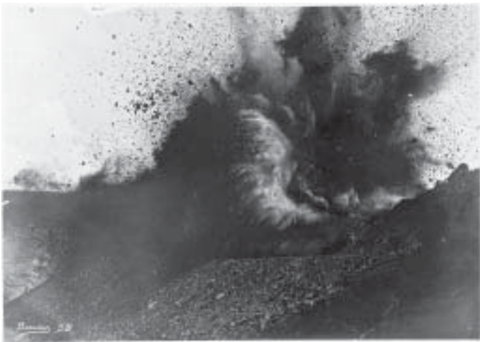
Explosion during construction of Elephant Butte Dam, c. 1910
