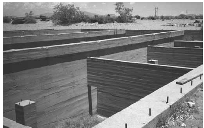
The only major artifact left from Camp Cody - the septic tank that was never used. Michael Kromeke Collection
