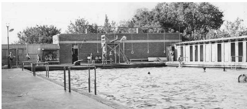
Deming's Army swimming pool. Funded by the Army and not completed until after the war, the pool provided faithful service from 1919 until the late 1990s. Deming-Luna Mimbres Museum Archive
