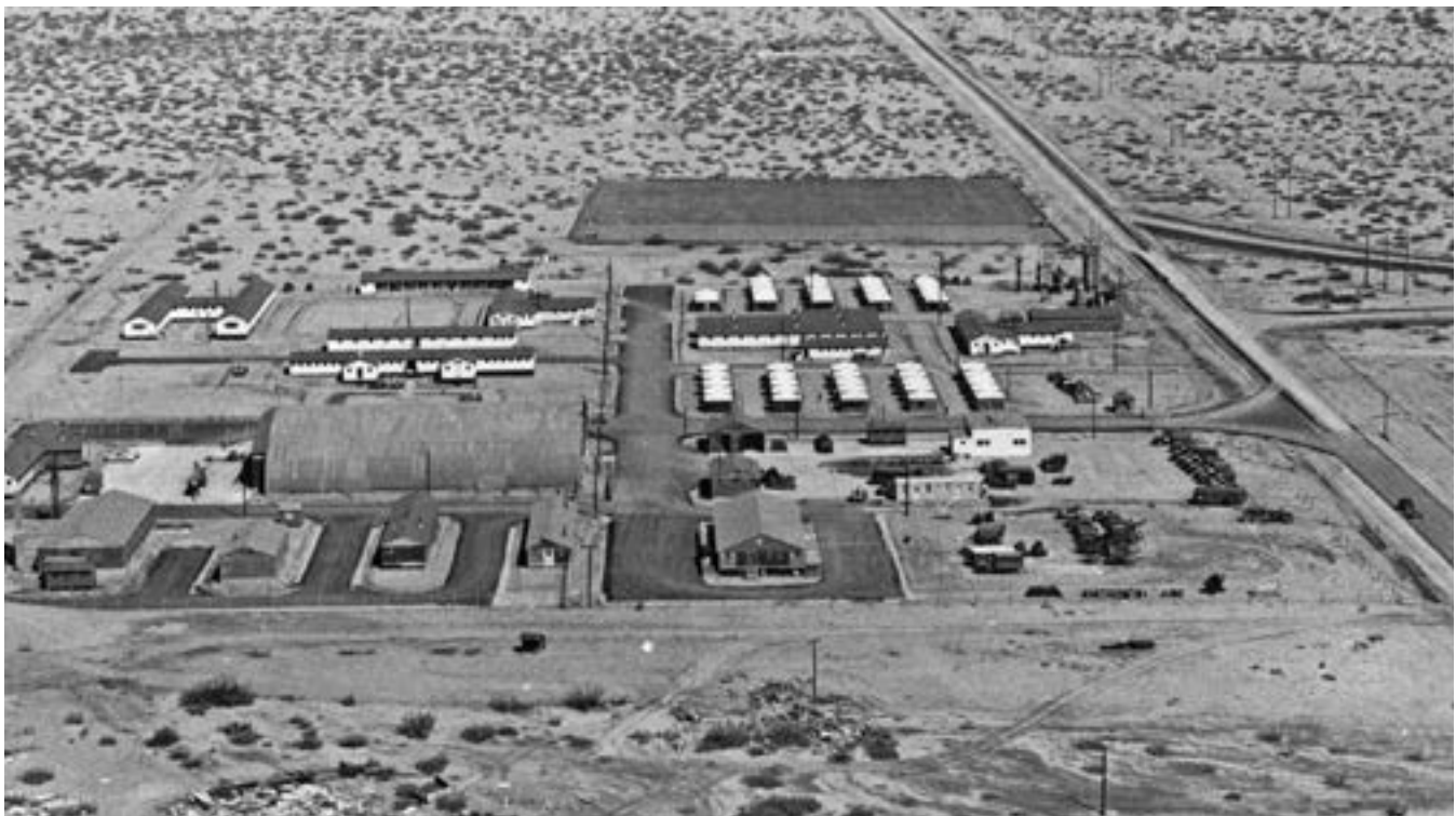
An aerial photo of the White Sands Proving Ground main post taken during the first week of August 1945. Most of the buildings were Civilian Conservation Corps structures from other parts of New Mexico that were taken apart and reassembled here. The only structure in this photo still standing is the old hanger, the large quonset hut, that was first used as the V-2 rocket assembly building. White Sands Missile Range Museum Archive.
