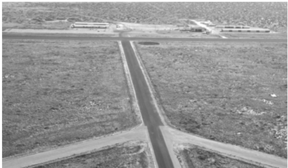
Aerial photograph of the West airport, circa 1968. (Image courtesy of Morris Drexler.)
