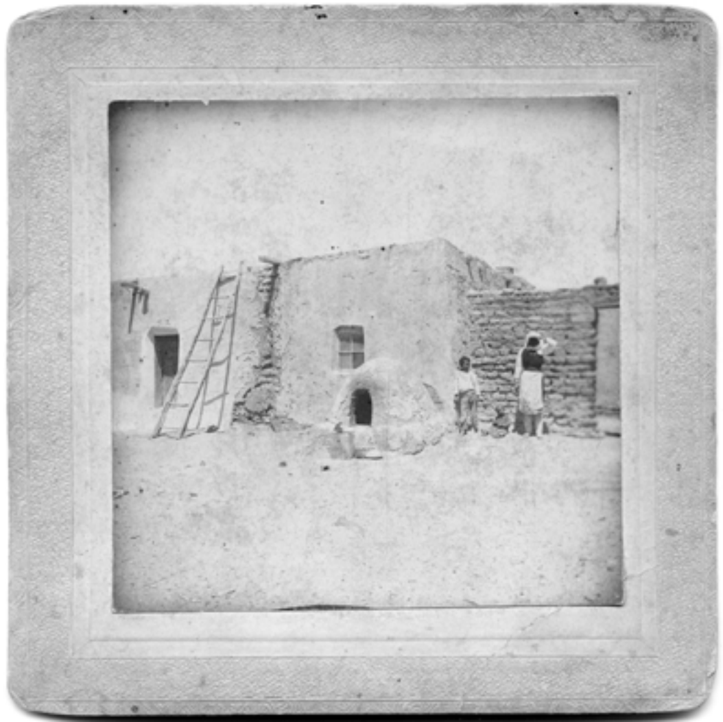
This image labeled as “Typical Mexican Dwelling” No. 1, Front, Las Cruces, N. Mex., 1900 is shown here with its mat. (Neale family photographs, RG2021-011-001)
