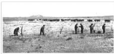
CCC construction of the Stock Driveway fence. Courtesy of the Palace of the Governors, #147671.
