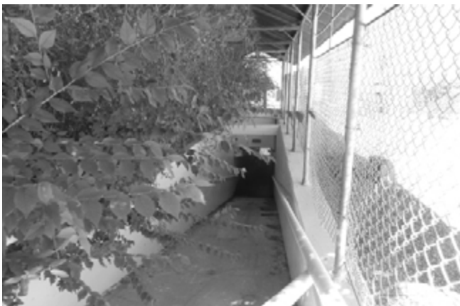
The tunnel connecting the two sides of town still exists today. Author's photo.
