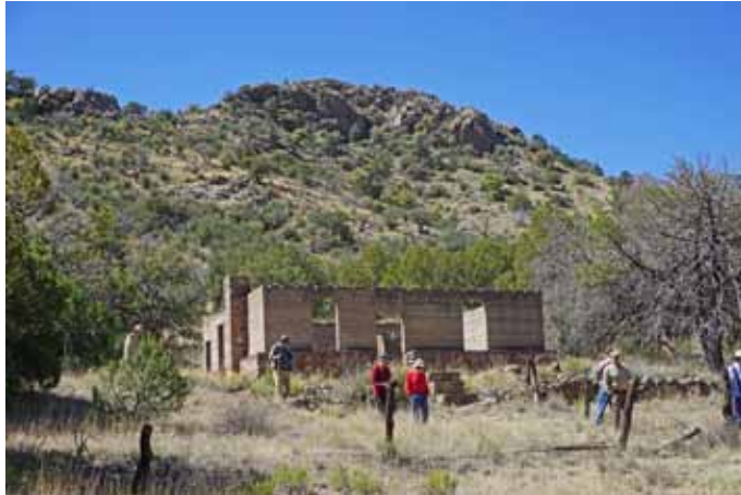
Main Beasley house.- poured concrete walls.
