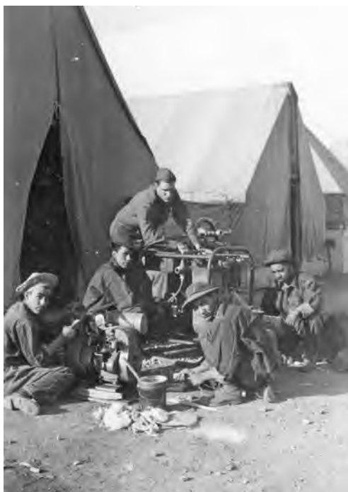
Preparing a water purification unit.
