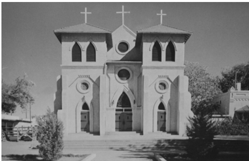
St. Genevieve's before demolition.
