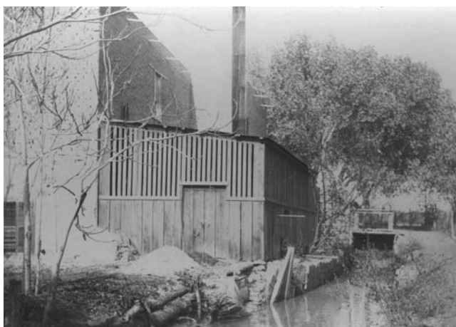
Figure 5. The Jacob Schaublin Mill was originally powered by the hydraulic power of the Acequia Genevieve (Photo from the author's collection).
