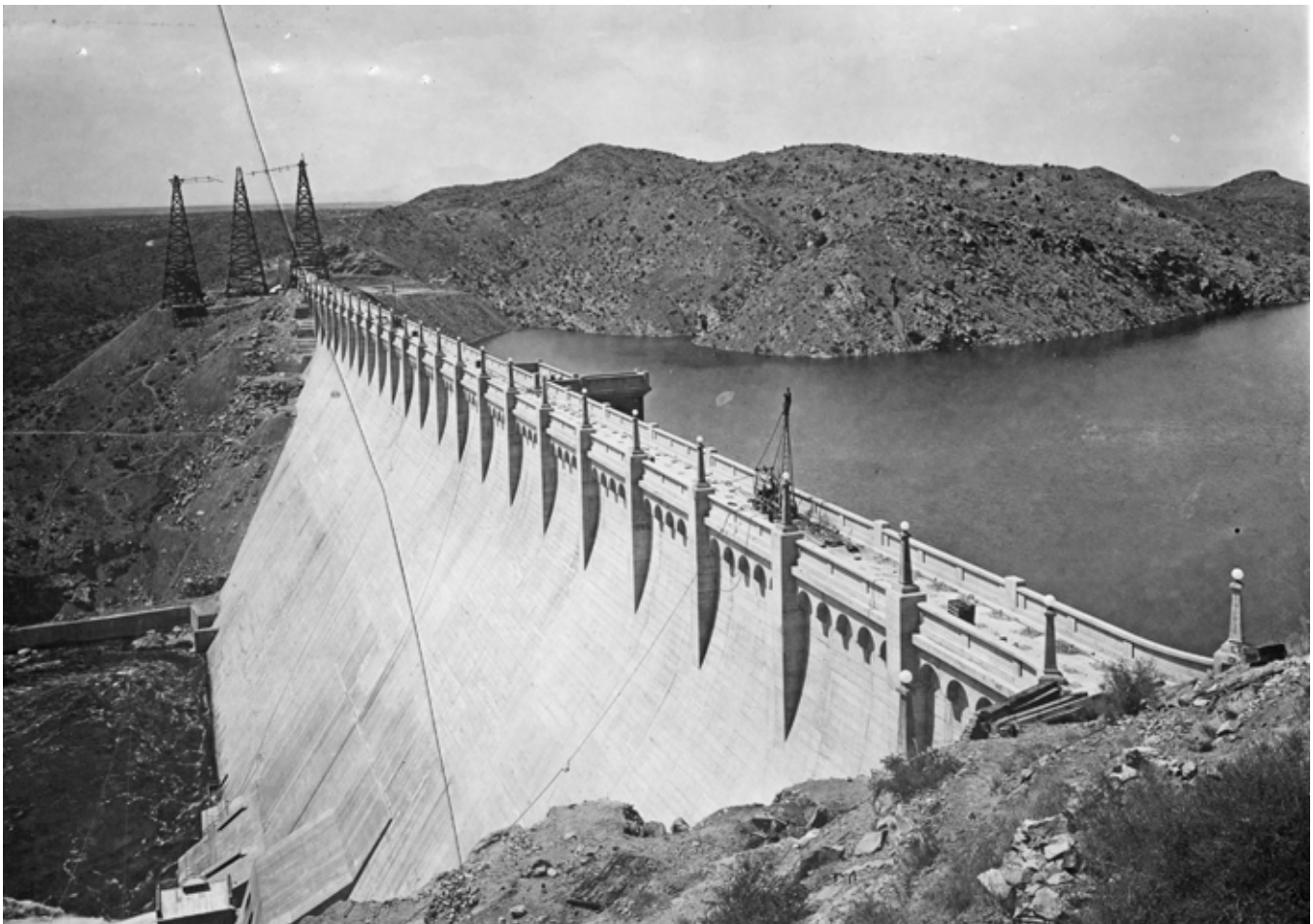
The completed Elephant Butte dam with a lake full of water behind it. At the time it was the world's largest irrigation dam, just over 300 feet tall. It was allowed to start filling in 1915.
