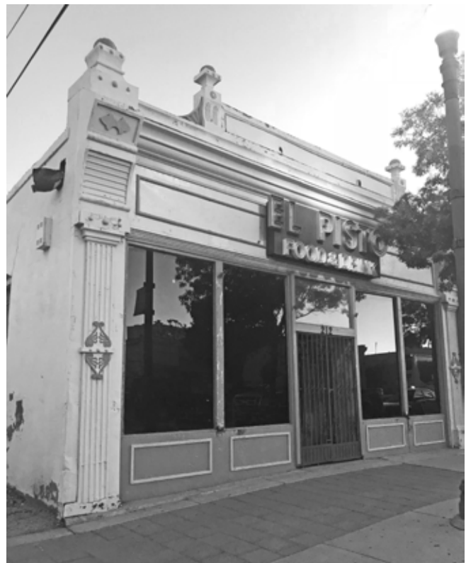
The building that once housed the Chinese laundry on Overland. Photo by the author.
