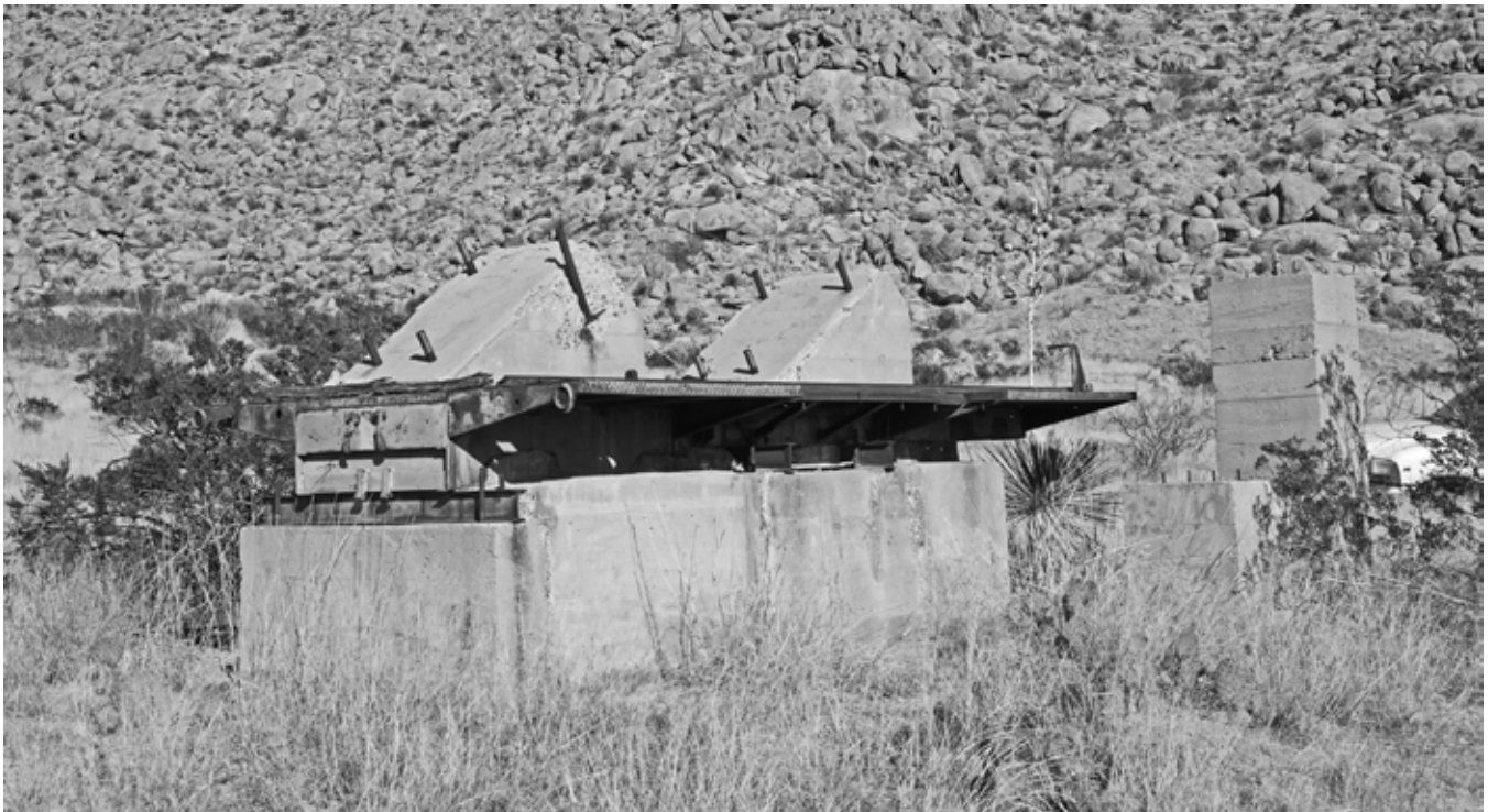
The concrete blocks at the Doña Ana Mountains site that held the meteor cameras. Photo by author.
