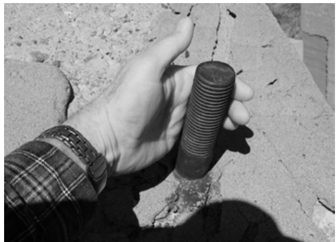
Bill Godby, White Sands Missile Range archaeologist, and I think this is the super-Schmidt camera mounted at the Soledad site. The unit weighed about 6,000 pounds so the foundation had to be bedrock solid so there was no vibration as the camera moved. The size of one of the bolts below testifies to the camera's weight.
