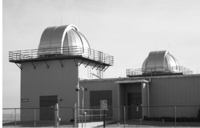
The front door to the GEODSS facility at White Sands Missile Range.
