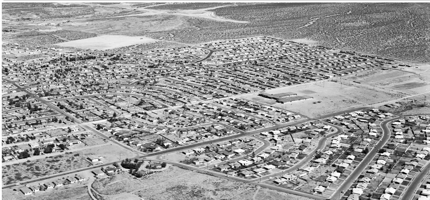
This is another image courtesy of Dr. Wallace. He estimates it was taken around 1960. It shows the big Bellamah development in Las Cruces, looking to the northeast. At the very top of the image you can see construction of the bridge for the intersection of Lohman and I-25, yet to be built. Also near the top is a large white square that must be the beginning of Young Park. The school in the middle right is Conlee.
