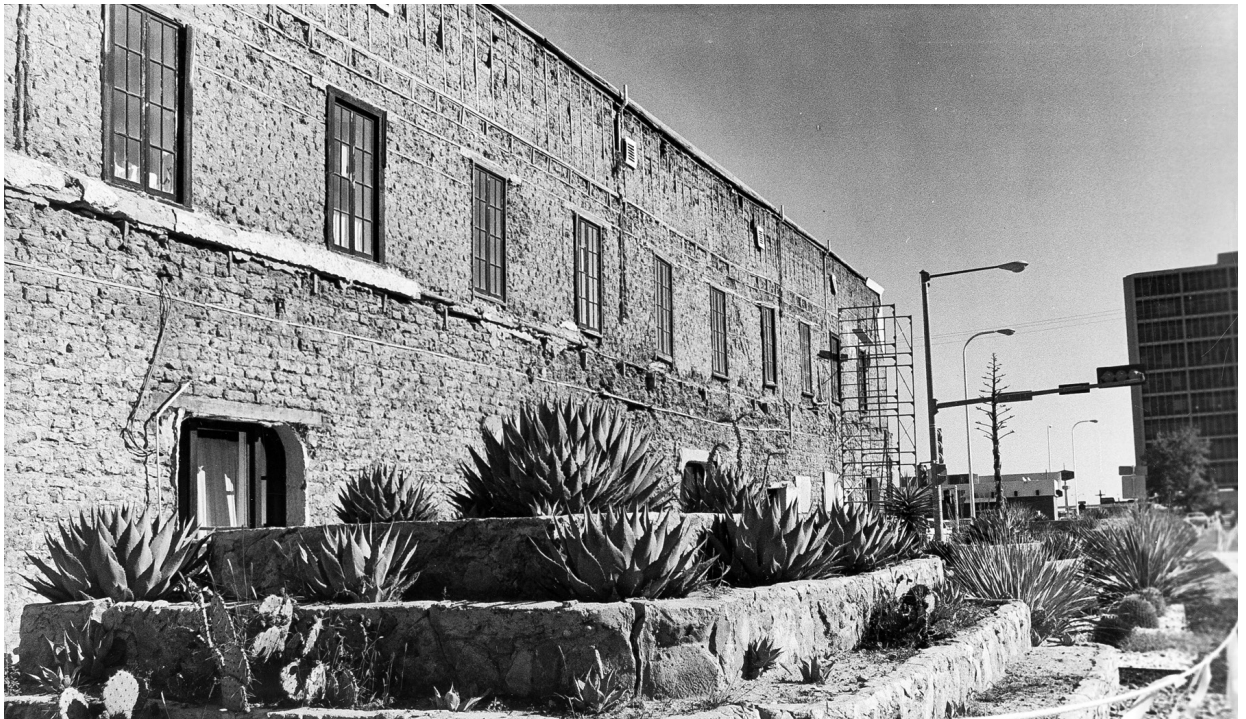
West elevation of the hotel showing the adobe structure under the stucco in October 1978. Photo by Jack Diven.
