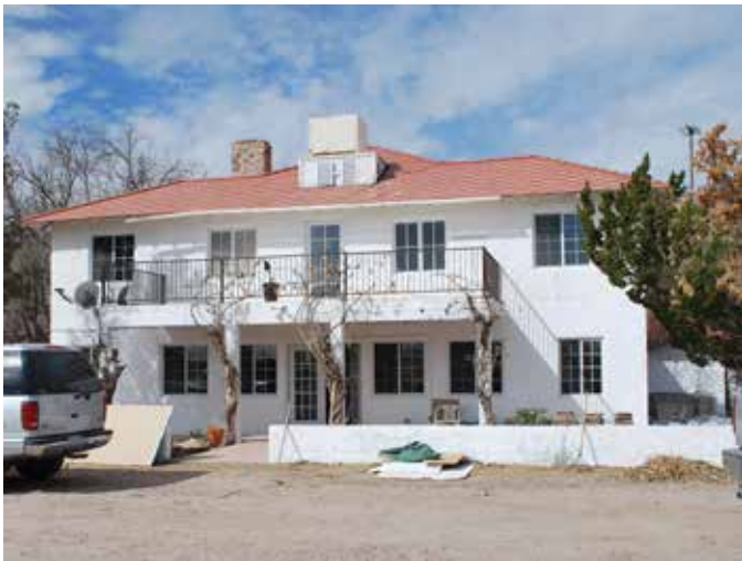
Current facility under renovation Photo by Bob Gamboa
