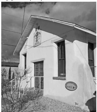
repaired with concrete, causing the adobes to retain moisture and the walls to crumble from inside out. The south wall in particular was unstable and it was clear the adobe bricks would have to be removed and replaced. By 2005, the entire building appeared ready to collapse.
